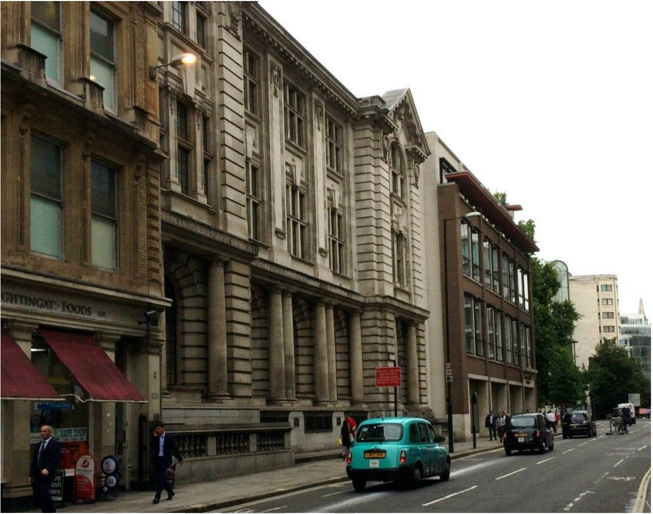
View 3 (grade II* listed retained stone façade)
